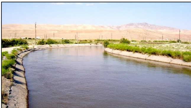
Fig 1: General view of the Samur-Absheron Canal. There are concrete slabs covering the bottom of this watercourse
