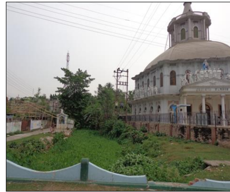
Fig 3: Concrete constructions on bank of river
