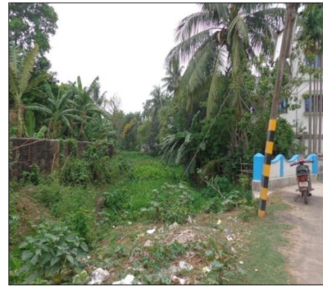
Fig 8: Manmade unscientific culvert
