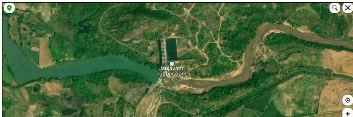
Jhanjavathi Rubber Dam 18.863573 N and 83.435136 E (Google courtesy)
